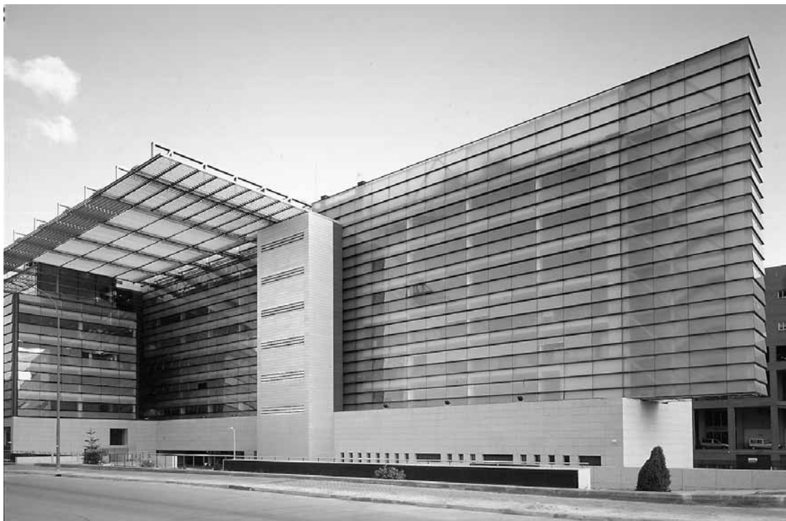
Vista general NO.
