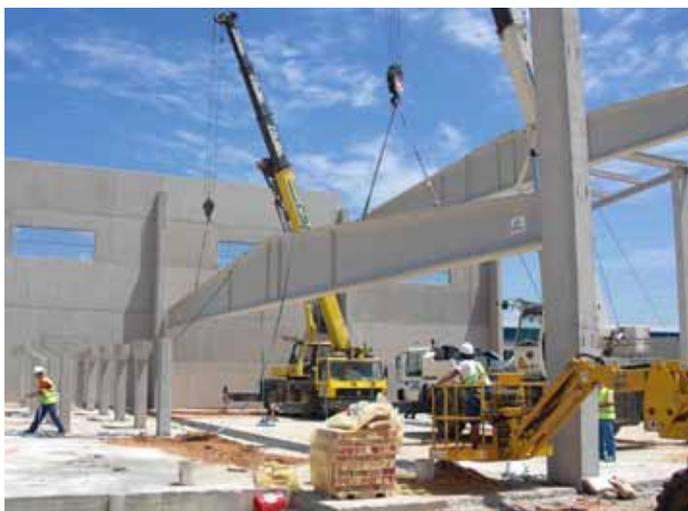
FIGURA 22 - MONTAJE DE NAVE INDUSTRIAL
