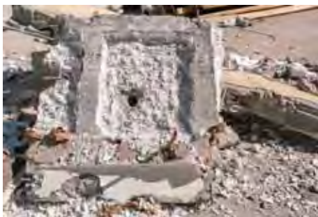
Losa de la azotea extraída. Slab extracted from flat roof.
