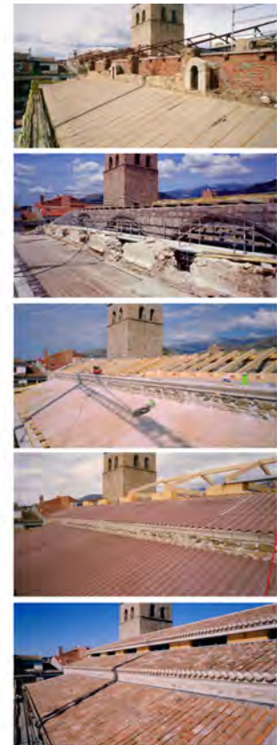
Roof assembly process
