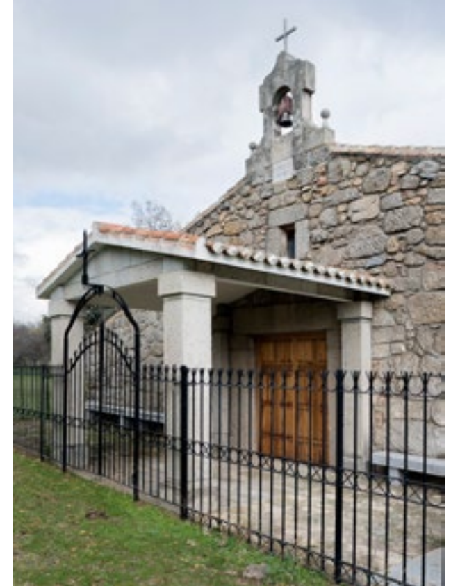
Facade of the Chapel of St. Michael Archangel, Navalagamella
