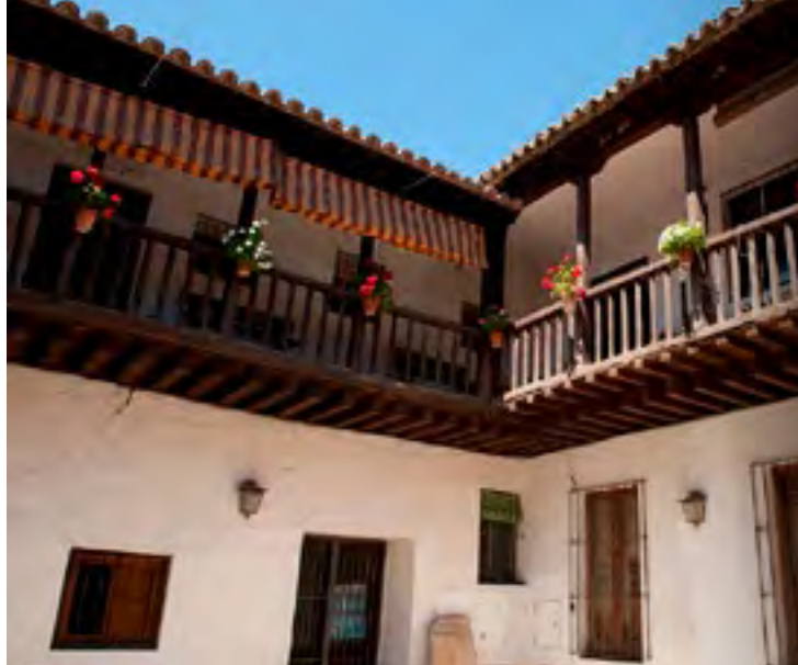
Courtyard of the old Antezana Hospital, Alcalá de Henares
